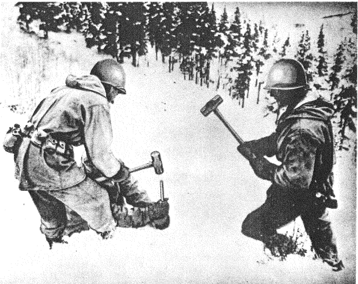
Figure 89. Three-man method of drilling holes in rock.
